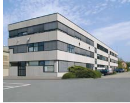
Carrier Lead Design Center in Germany
